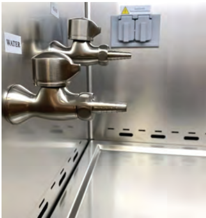
Water and Gas Taps
